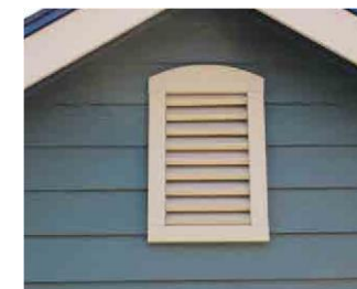
Large Gable Vent
