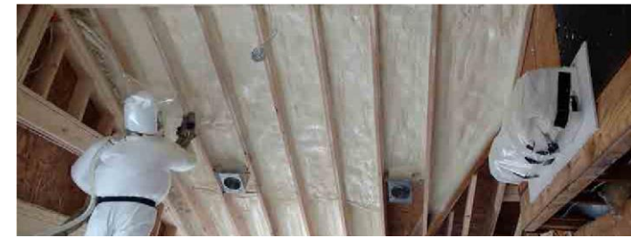
Spray Foam Insulated Floor
